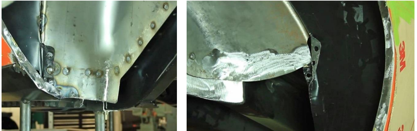
Figure 40 - Weld Outer Wheel Tub Flanges
