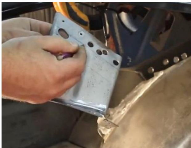
Figure 43 – Trim the Trunk Hinge Reinforcement
