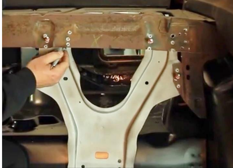
Figure 9 - Drill Out Spot Welds
