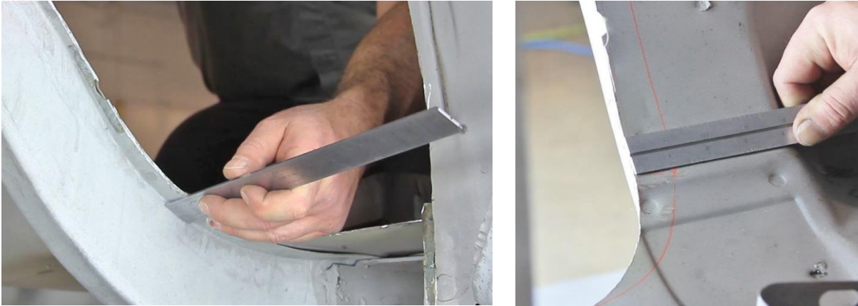
Figure 18 - Transfer Flange Dimension
