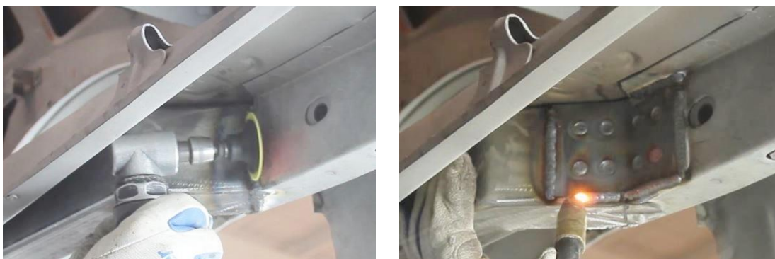
Figure 23 - Weld Inside Frame Rail Doubler Plate
